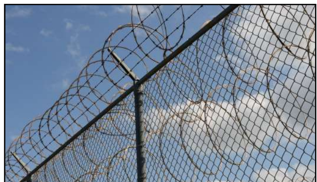
CHAIN LINK FENCING WILL LINE THE CAMPUS PERIMETER.
